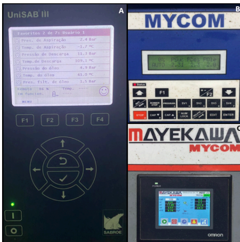
Figura 30 - IHM compressores. (A) Sabroe, (B)/(C) Mycom.
